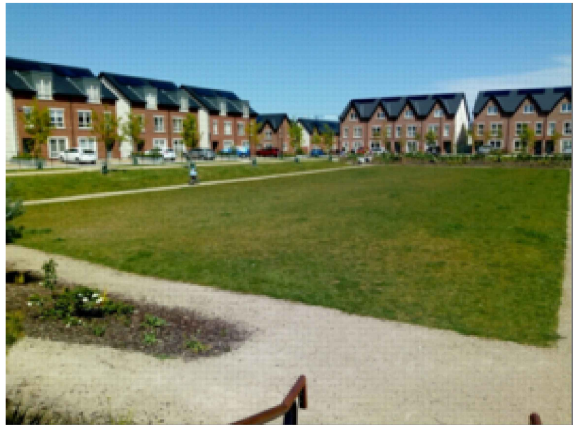
IMAGE 002 - OVERGROUND DETENTION BASIN EXAMPLE - PHASE 1 GRAYDON DEVELOPMENT
